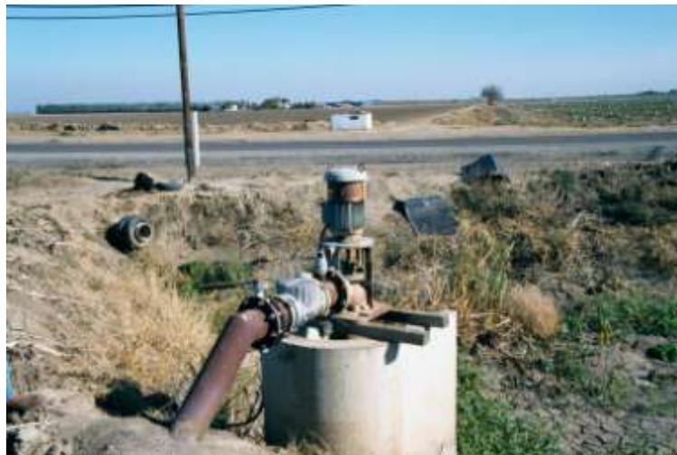
Figure 4. Control (butterfly) valve, air-vacuum relief valve, and check valve located downstream of tailwater return pump.
