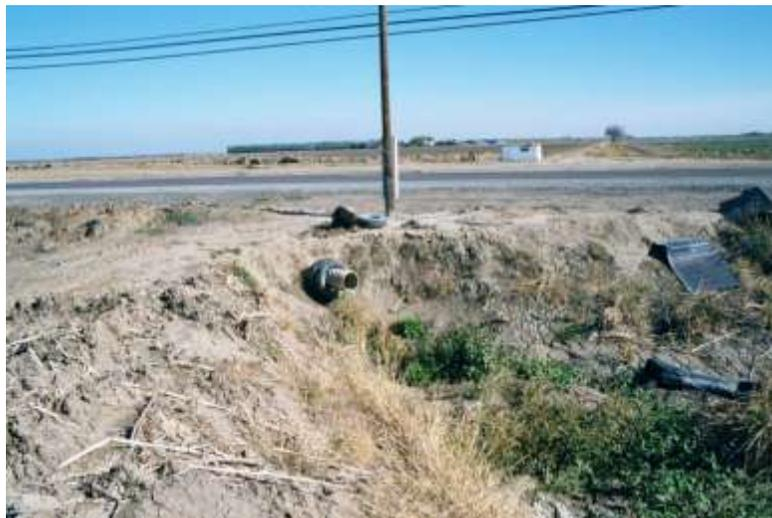
Figure 2. Cantilevered pipe discharge into tailwater pond.
