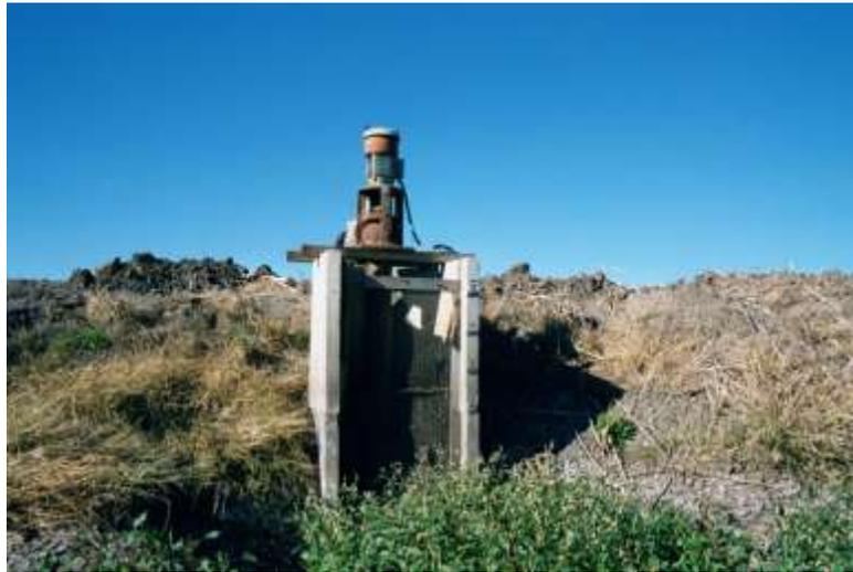
Figure 3. Trash screen on a concrete sump intake box.
