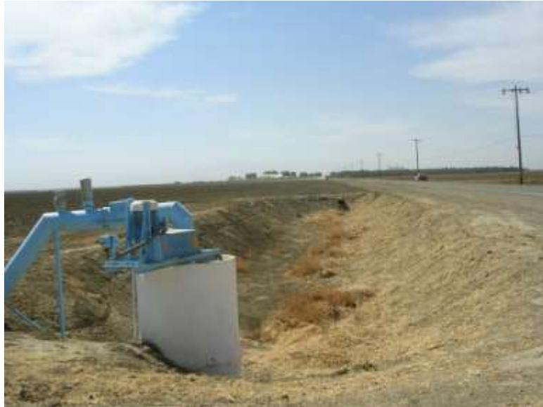
Figure 1. Tailwater collection system.
